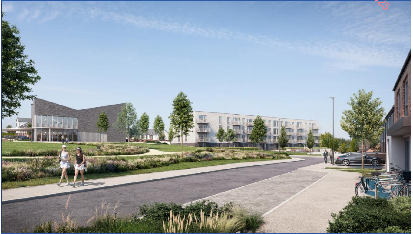
Figure 2.16: CGI Community Building (LHS)
